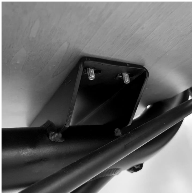
Picture 23 - Cargo box screw connections - bottom side
